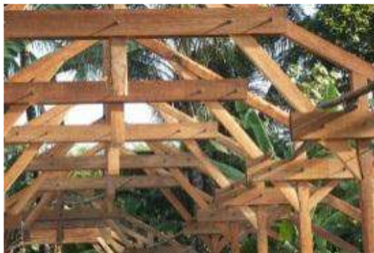
Image 24. Wooden truss joined with 12mm bolt. The ventilation for cooling down the building structure
