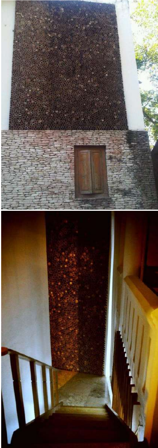
Image 39. Bamboo Used as Wall Covering on Some Parts of the House (Indoor and Outdoor) Source: Eko Prawoto, 2013
