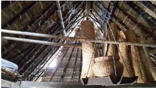
Image 6. Traditional Lombok house roof structure
