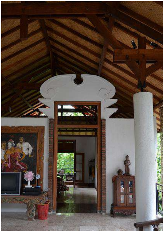
Image 37. The Main House' Structure Adapted Traditional Thatched Roof Completed with Traditional Ornaments.
