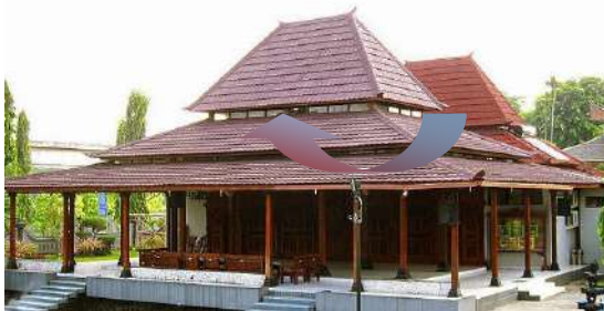
The wind goes inside the building through the roof gap
