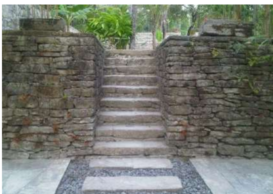
Image 34. Natural Stone Used for Pedestrian Way Along the Site Source: Eko Prawoto, 2013
