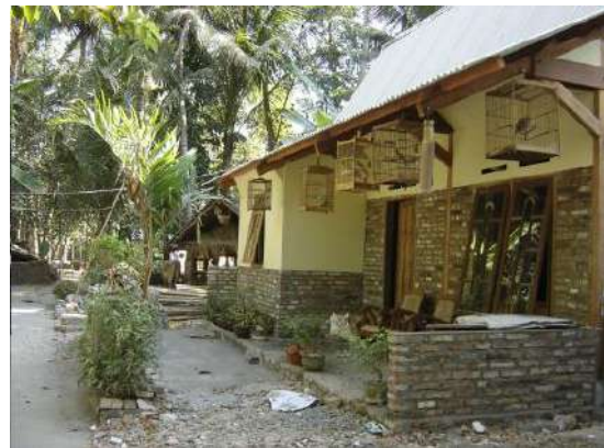
Image 23. The inclined roof used in order to avoid leaks when it rains and the overhangs designed to protect the house from direct sunlight
